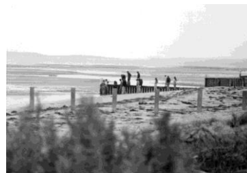
Groynes at east Silverleaves 1967
